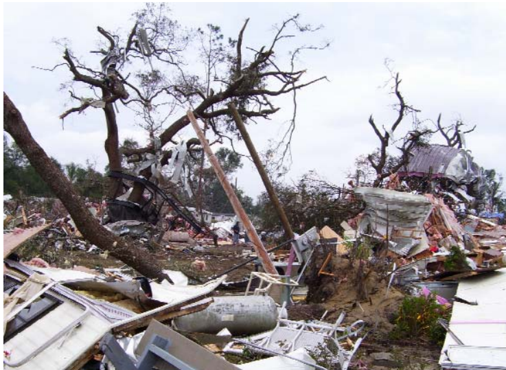
Aftermath of Tornado at Sunshine MHP near Lady Lake, Florida
